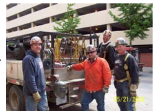
Above: Shane Ricks, Charlie Roberts, Brandon Forar & Ted Desantell after a Sunday shift on the Heart Hospital Skyway Project.
